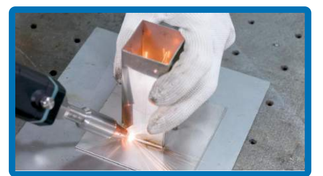
Square tube welding
