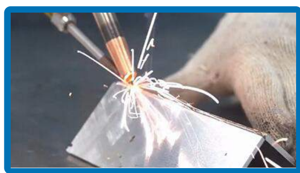
Outside fillet welding
